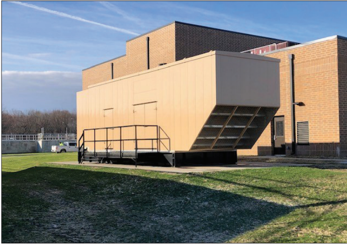
2nd page top left: Weather resistant enclosure, designed to meet a specific footprint for a waste water treatment plant.
