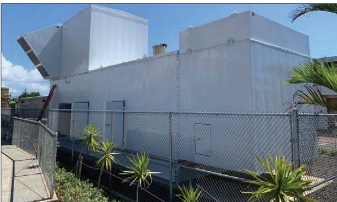
Acoustic enclosure for a CAT C175-20 rated at 3900 kW. Large UL142 fuel tank and sound rated for 73 dBA @ 7 meters.
