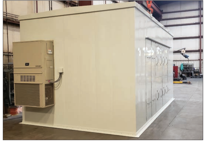
Climate controlled electrical E house with 15 kV paralleling switchgear.
